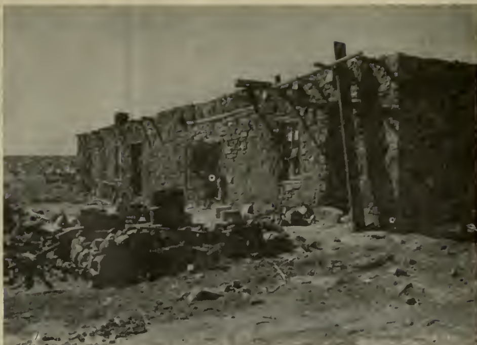
Three Spanish-American families live in this house, which is of red stone, not adobe
